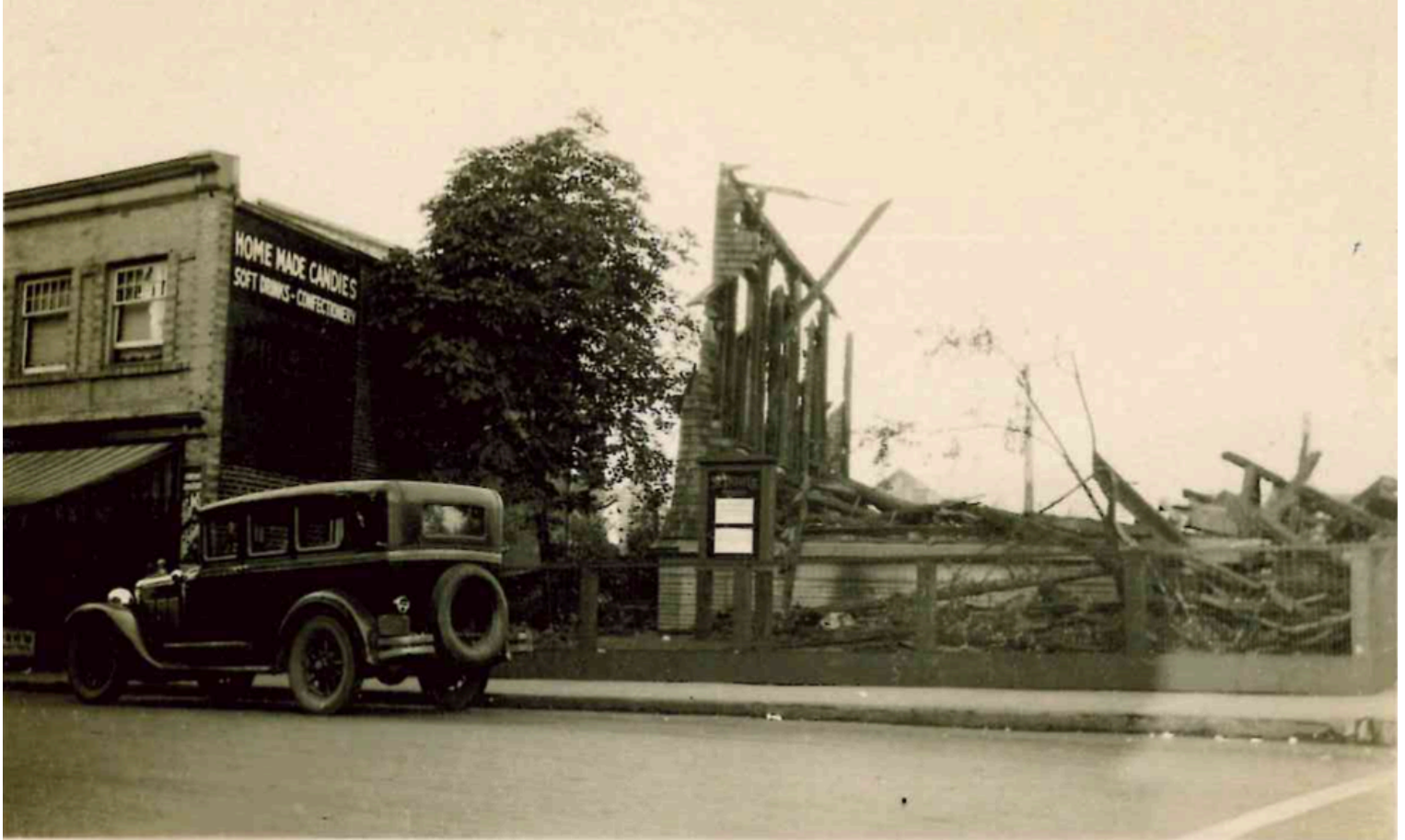
The aftermath of the fire
