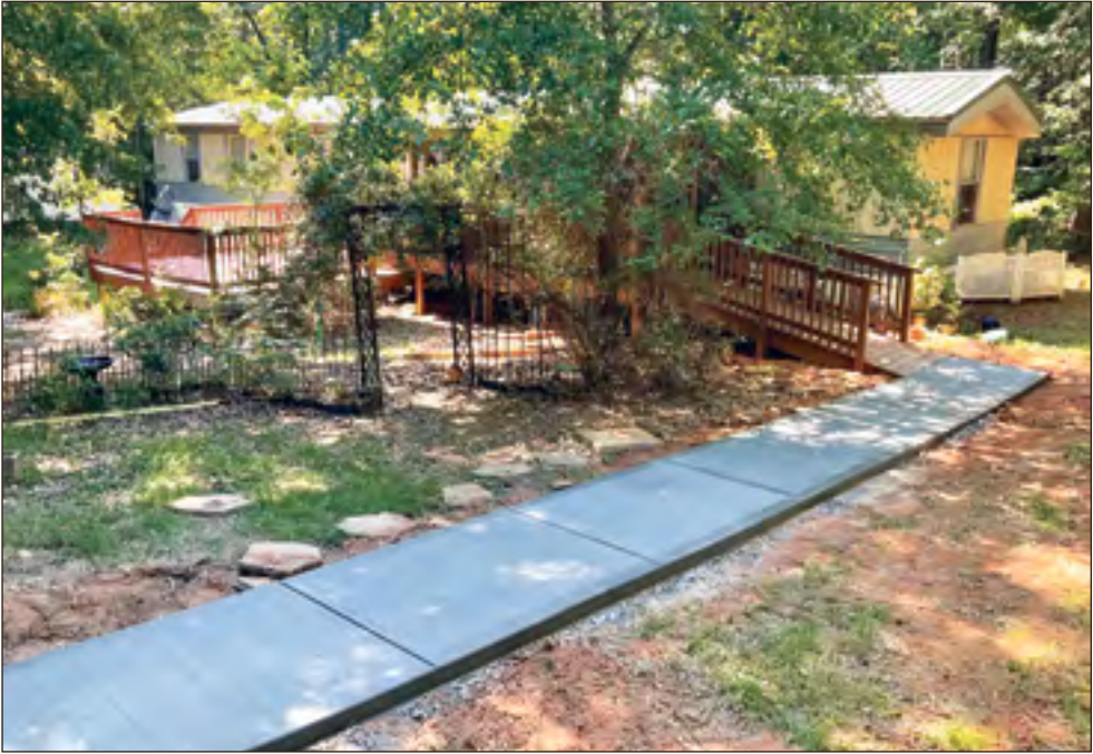
They also were able to build a wheelchair-accessible ramp for his wife and construct a small sidewalk going from the ramp to their car so the couple can get out easily for doctor visits.
