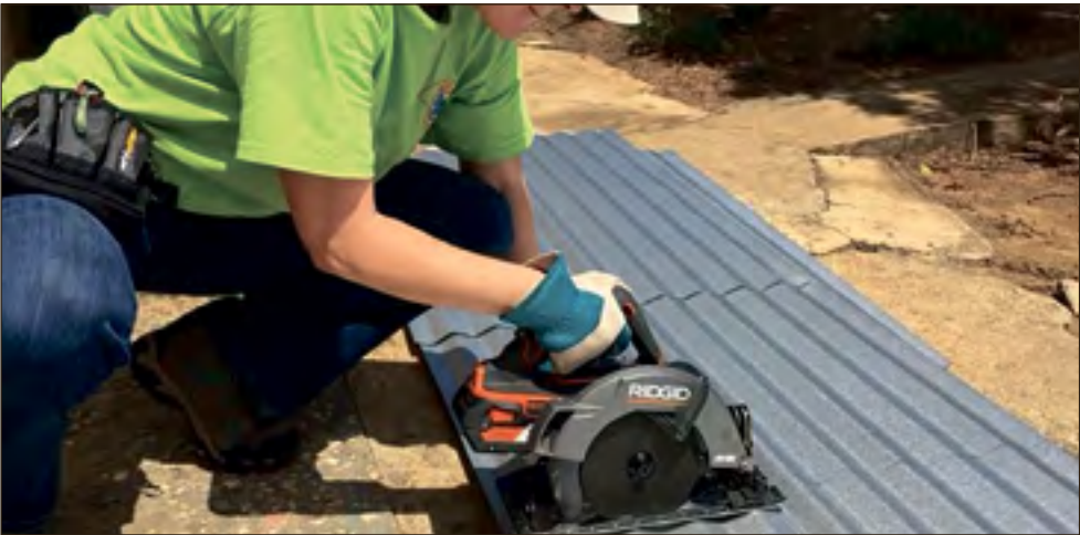
Here, an UMVIM volunteer works on a home in Puerto Rico damaged by a hurricane.
