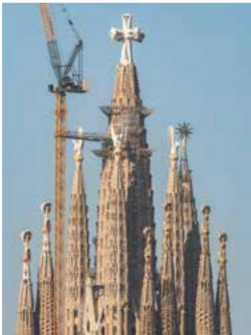
THE INTERIOR AND EXTERIOR (under construction) of Sagrada Familia in Barcelona, Spain.
