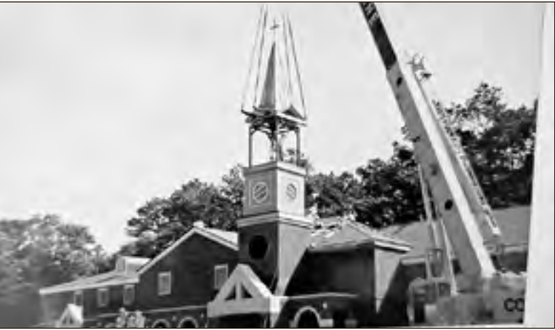
The steeple is lowered onto the enlarged church building in 1991.
