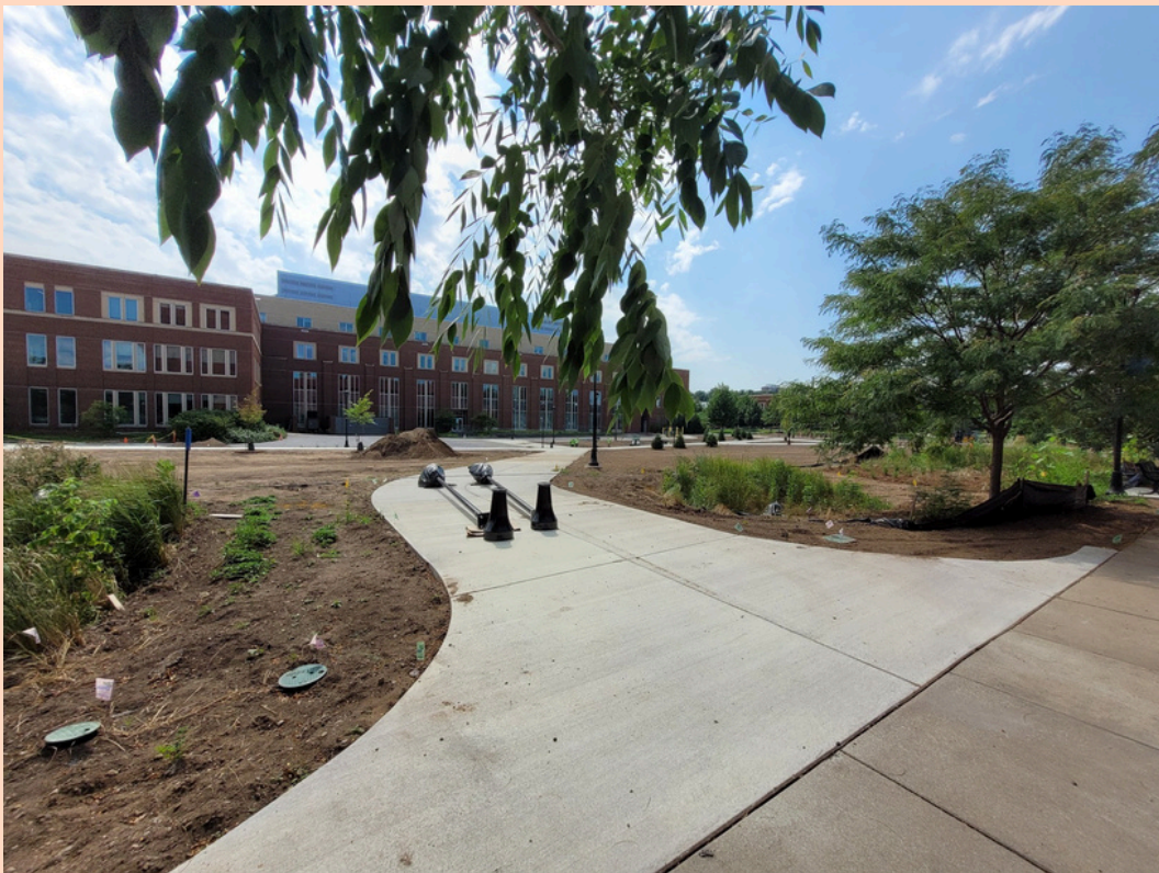
The former site of Zorn Arena, Kjer Theater, and Brewer Hall is shaping up nicely for greenspace at the campus entrance. (It's also hiding lots of underground infrastructure put in this summer for Hibbard Hall.)
