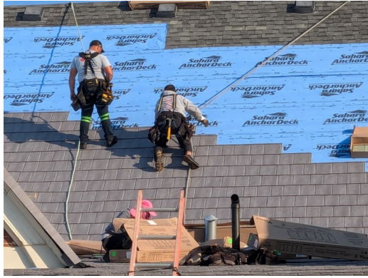
Installing New Roof (above)
