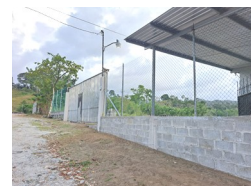
The completed wall and fence in front of the church property.
