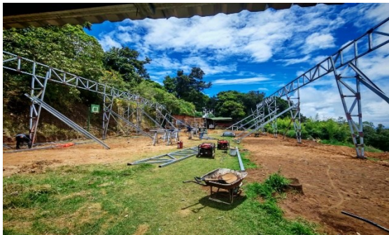
Construction at the Coronado Camp
