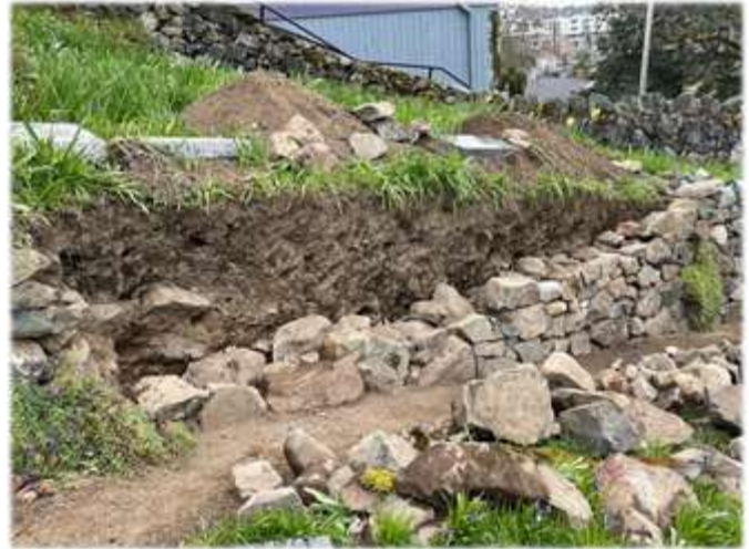
The dry stone wall being rebuilt Photo credits for pictures on page 23 and 24: Barb Prescott
