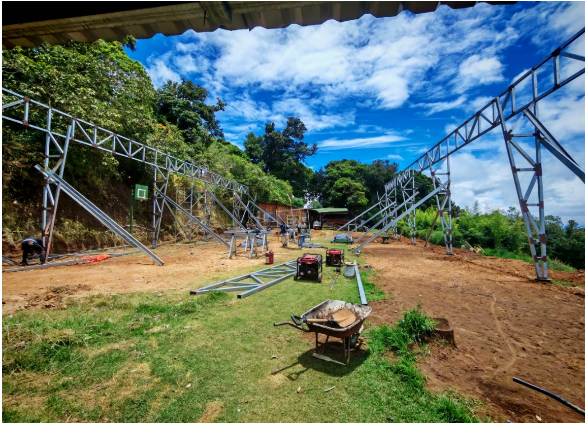
Construction site at the Coronado Camp in Costa Rica
