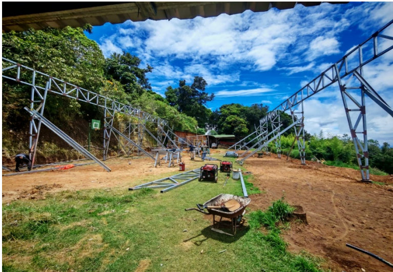
Construction site at the Coronado Camp in Costa Rica
