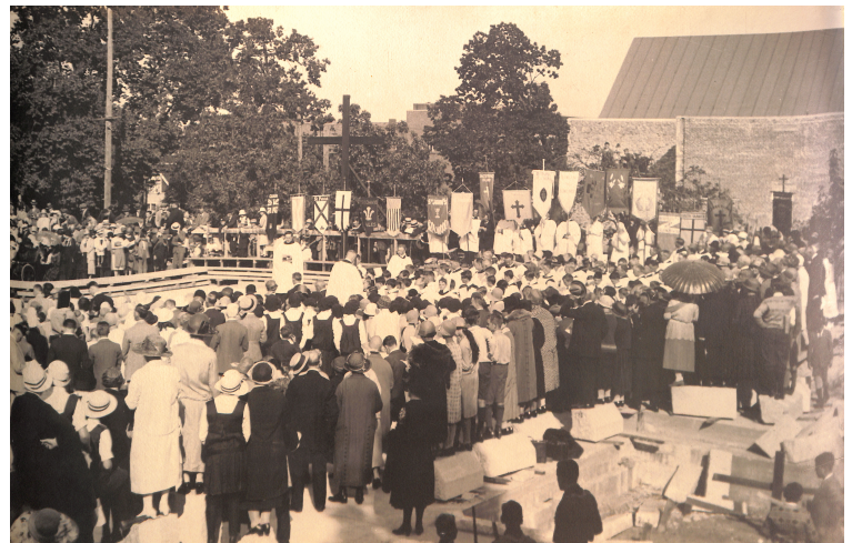
Laying of cathedral foundation stone, March 21, 1927 (Ph. 208)
