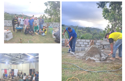
Starting work on the back wall.
