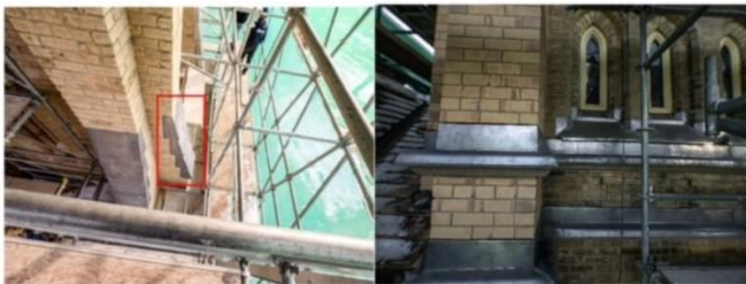
Metal work on tower
