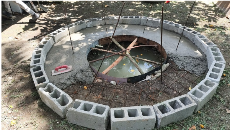
Framework for the well under construction for the church area in Finca 51
