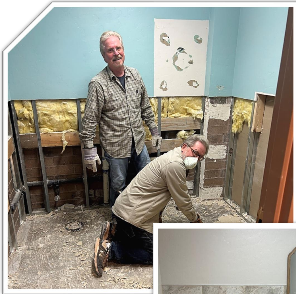
The Upgrade of One of the Narthex's Bathrooms Has Begun
