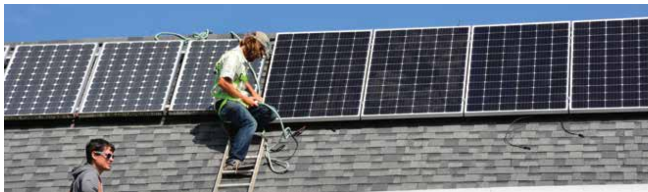
Installing the solar panels September 2018. PHOTO Margaret Peake
