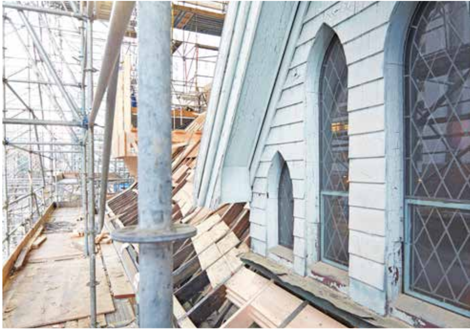
Reattaching the roof dormer. PHOTO Martin Knowles of MKPhotomedia
