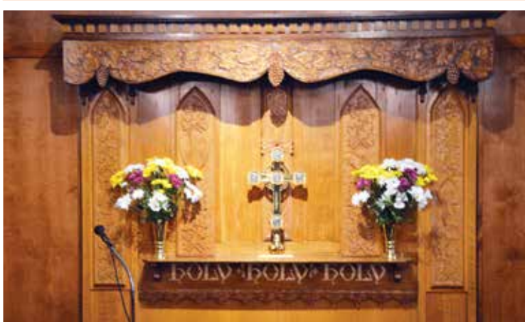
The reredos, damaged in the fire is beautifully restored complete with the refurbished hand-lettered, gold painted "Holy Holy Holy" and all set against the brand new wood paneling.
