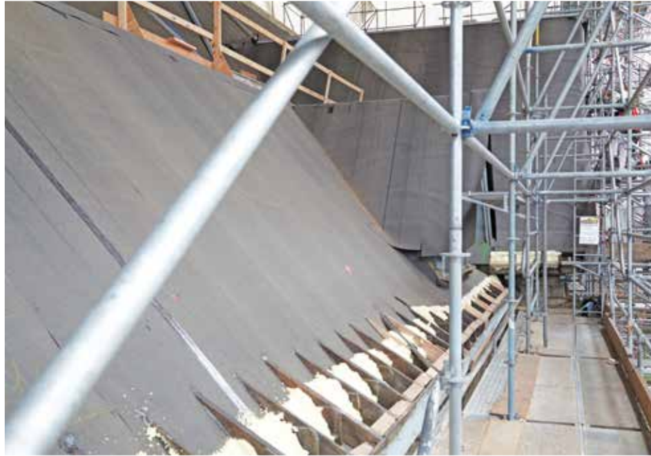
Completion of insulation and the vapour barrier. PHOTO Martin Knowles of MKPhotomedia
