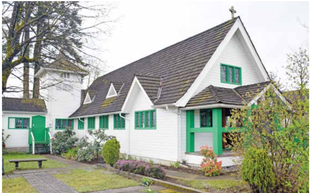
The church exterior facing southeast.
