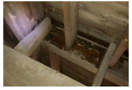
part of the top plate on the southeast corner of the bell tower, repair any roof damage and replace all of the shingles on the steeple above and below the bell.
