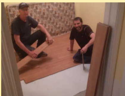
Mikko & Dan laying flooring in Fort Severn church parsonage
