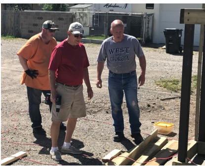
Roger Cole, Tom McIntyre & Don Koch building the garbage enclosure
